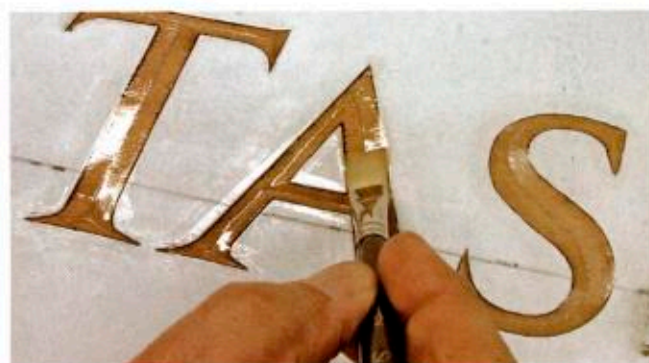
After having dusted the letters with kaolin powder and vacuumed away excess, Francis applied LeFranc Charbonnel's 24-hour, slow size to prepare them for gilding.
