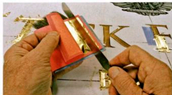
Francis used a gilder's knife to cut partial 23k-gold sheets, which he said was less awkward when applying goldleaf to intricate surfaces.
