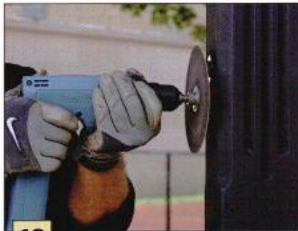
12 We then smooth out the saw cut with a cordless grinding wheel.
