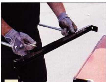
7 In the milling phase we had hand-routed a recessed edge on each end-grain of the panel to accommodate the channeled bracket that will hold the panel to the posts.
